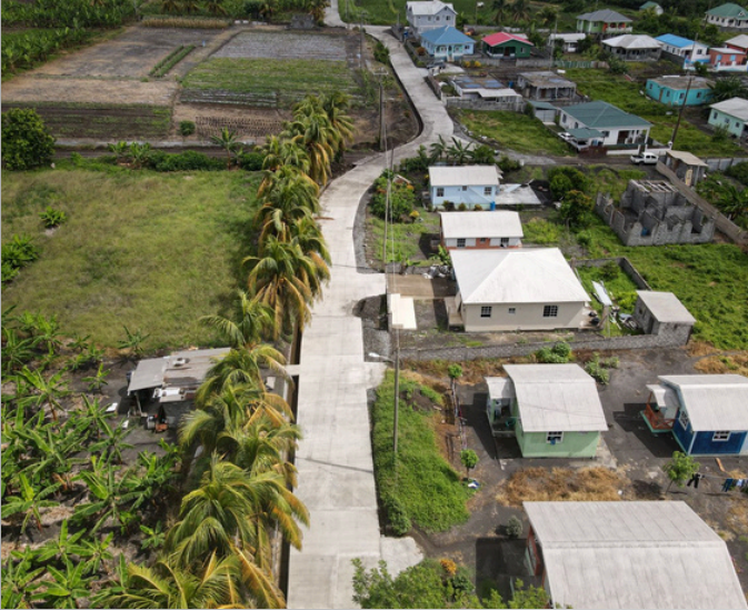
LANGLEY PARK FEEDER ROAD
